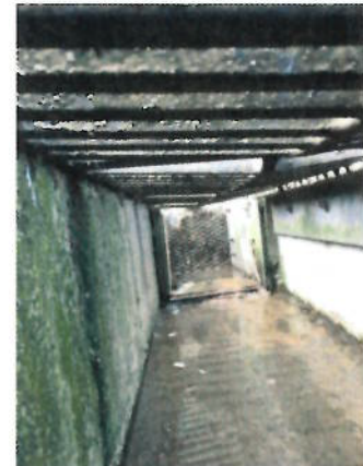
Trench drain after filter, all clean!
